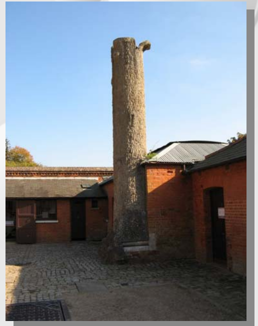
Figure 6 - A concrete tree – the chimney of a gas works! An early form of being environmentally friendly.
