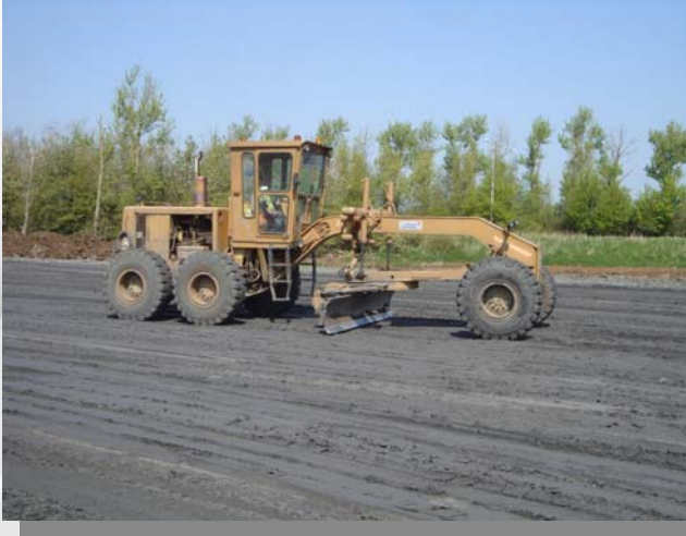
Figure 8 - Compacting PFA on the M4, Jnc. 11.
