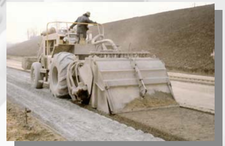
Figure 4 - Making a Fly Ash Bound road base
