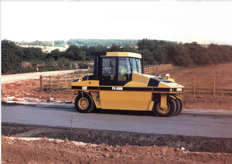
Figure 1 - Gotham by-pass, Notts. Compacting CFA.
