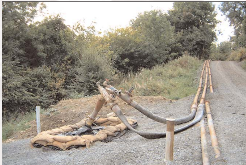
Grout injection point
