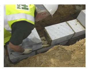
The compressive strength of Aircrete, as tested in accordance with BS EN772<sup>b</sup>, ranges from 2.9 N/mm2 to over 9.0 N/mm2, depending on density. This satisfies the structural requirements of a wide range of building types. The drying shrinkage of Aircrete is tested in accordance with BS EN680.
