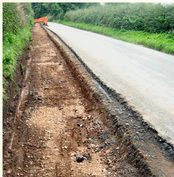
**Figure 2 - Road reinstatement using FABM**
