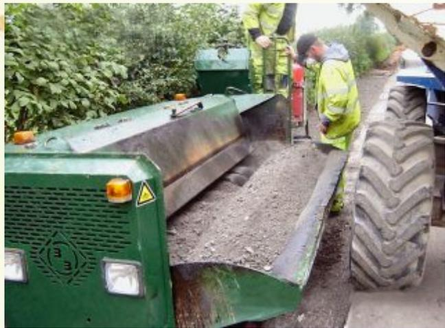
Figure 3 - Placing lime/fly ash based FBM1 HBM
