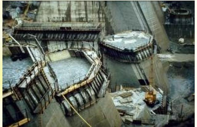
**Figure 5 - Dam construction using fly ash concrete in the USA**
