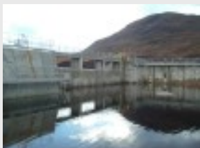
Figure 4 - PFA is used in concrete to enhance durability
