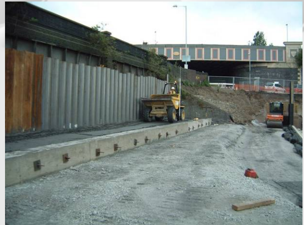
Figure 3 - PFA used as a reinforced earth embankment
