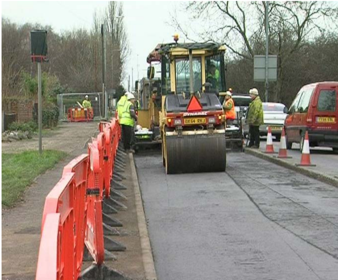
Figure 1 – Laying FABM 1 in Staffordshire
