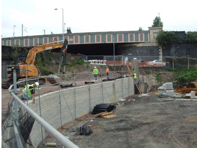
Figure 1 – a reinforced earth PFA embankment
