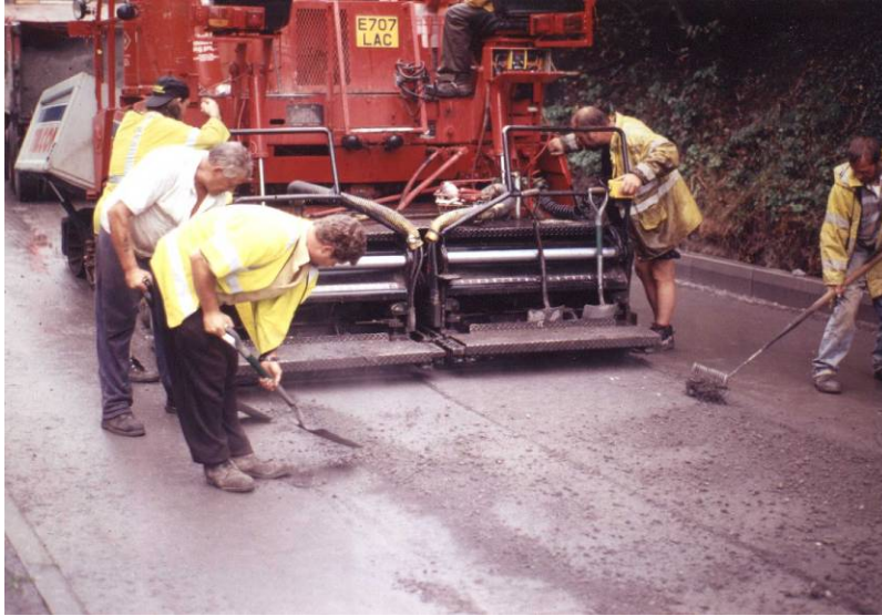
Figure 2 - Laying FABM on the A52
