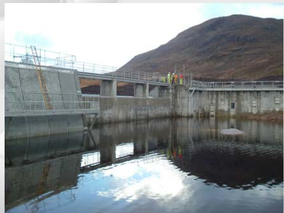
Figure 1 - A fish pass and slipway made using fly ash concrete
