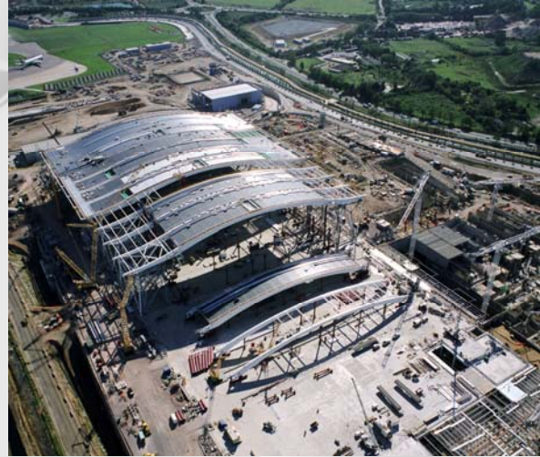
Figure 2 - Heathrow Terminal 5 used fly ash concrete
