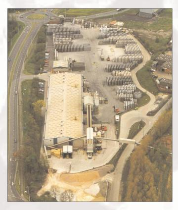
the pallet to a storage area for curing. Commonly this curing area consists of enclosed chambers that are heated at temperatures up to 80C, depending on the heat source, to accelerate the cement hydration and strength development to optimise the throughput of the plant. Blocks are then packaged into cubes of various configurations and further stored in a stockyard if required to achieve the final strength.
