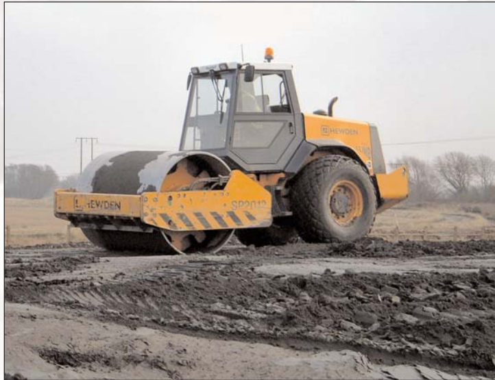
Figure 3 - Compacting PFA on the Selby by-pass
