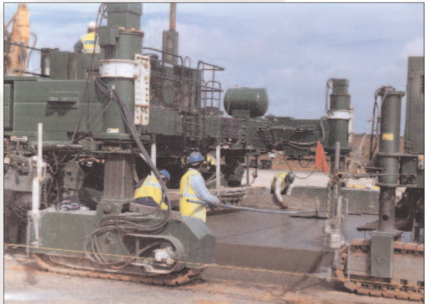
Fly ash concrete being used on East Midlands Airport taxiways (courtesy of Fitzpatrick Contracting Ltd)
