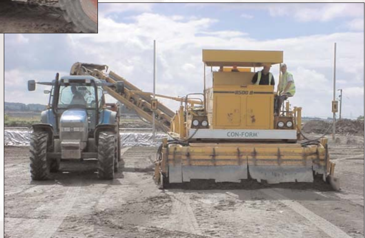
Final trimming of CBM
