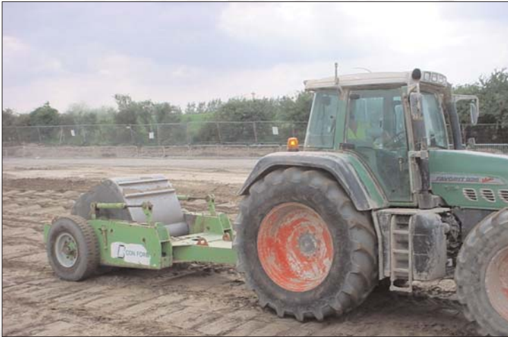
RDC to induce initial settlement
