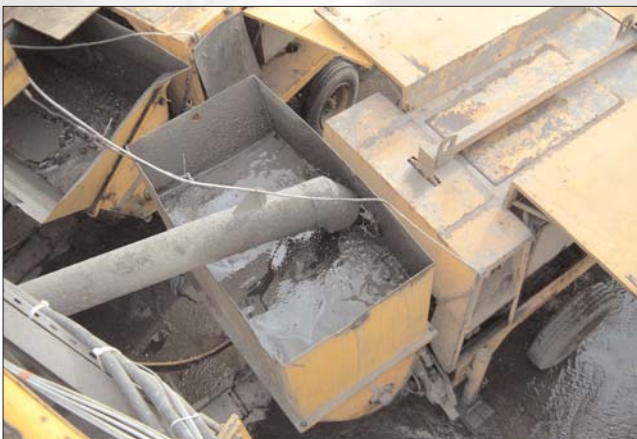
Figure 3 - The grout entering the Schwing pump
