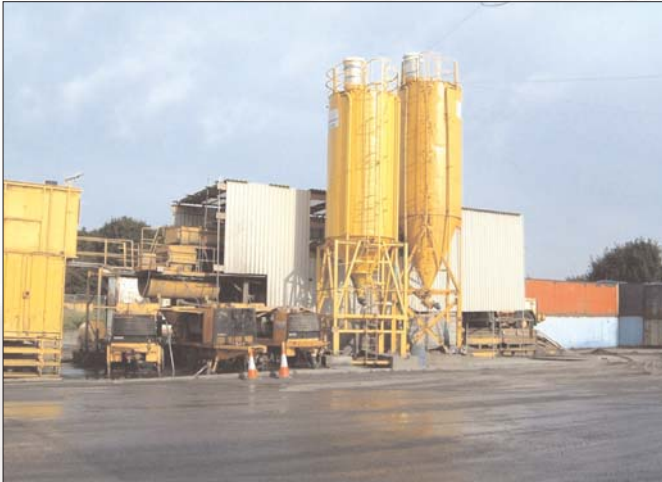
Figure 1 - The Mons Hill grout production plant
