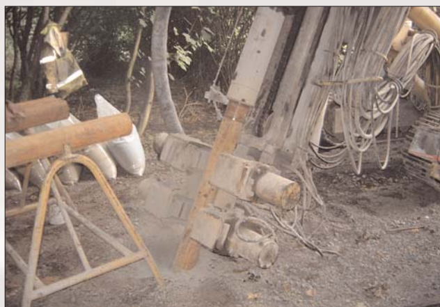
Figure 5 - Drilling the injection holes
