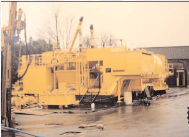
Figure 4 - The dust free 'Groutmaster' plant
