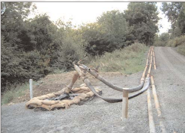
Figure 6 - One of the grout injection points
