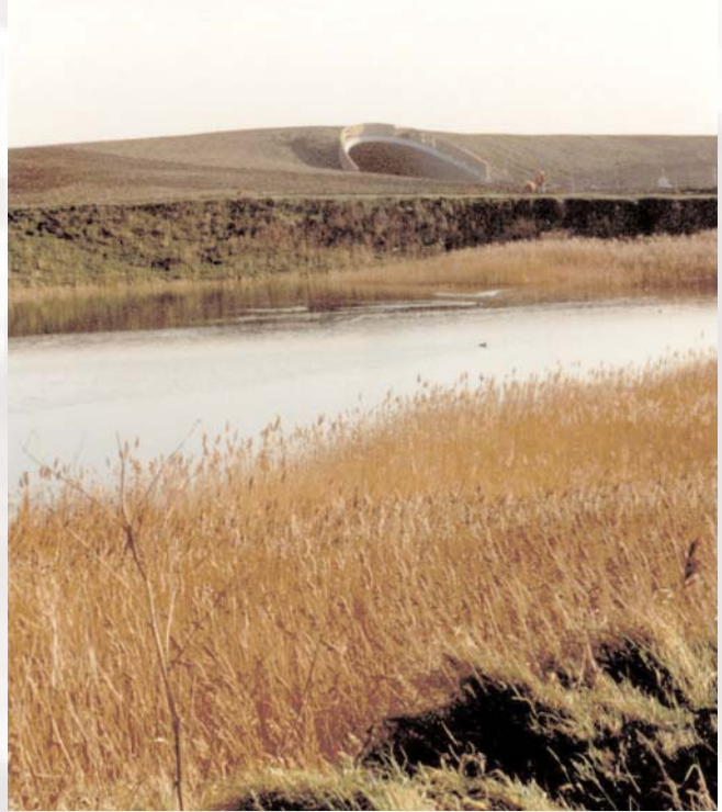
Access bridge over the railway near Burry Port
