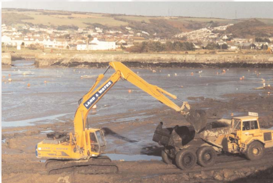
Removing the silt from Burry Port harbour
