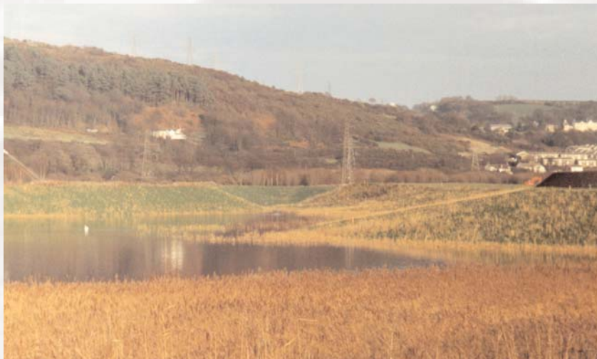
A pool created using fly ash as a fill material
