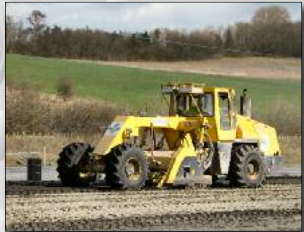
Figure 5 - Rotovating the cement into the fly ash/lime mixture
