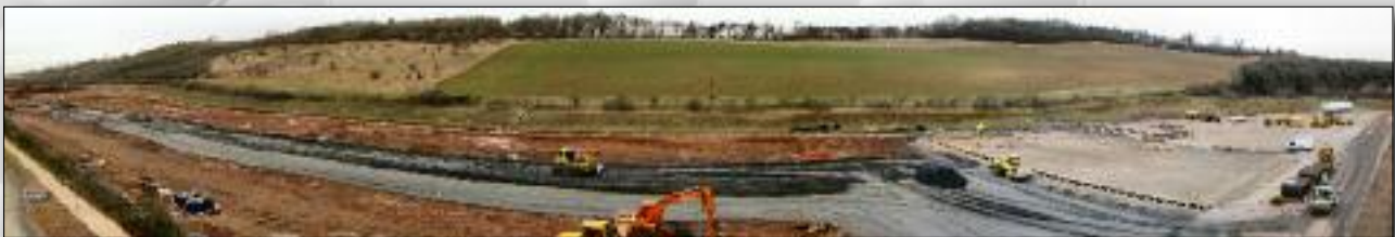
Figure 1 – Panoramic view of the Construction Laydown Area
