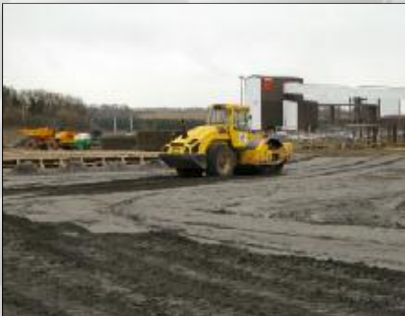
Figure 6 - Compacting the FABM 5
