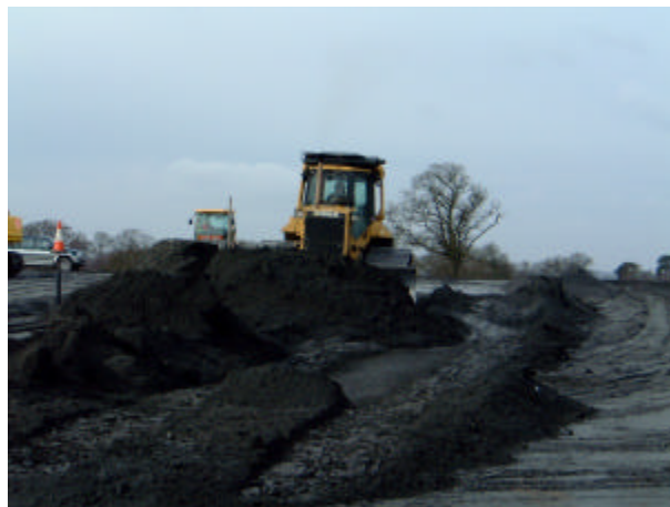
Figure 2 – Will the use of PFA of as a fill material become too difficult for contractors?
