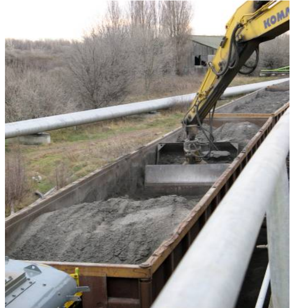
Figure 2 - Unloading 2000 tonnes of PFA a day at Northwich
