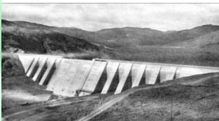
Lednock Dam - one of the first applications of fly ash in concrete once!
