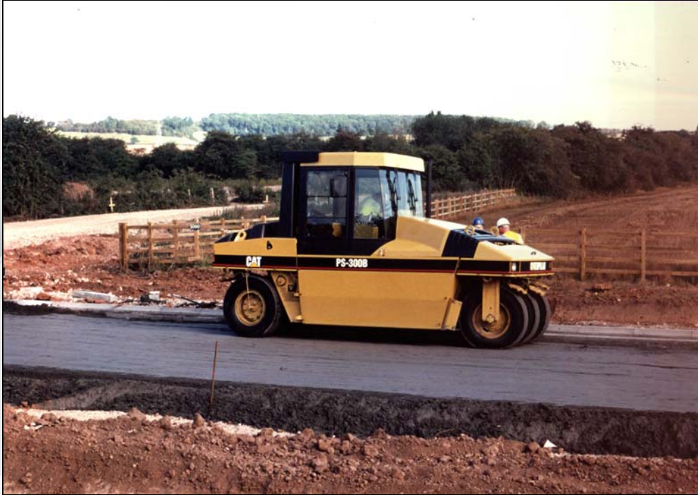
Figure 2 - Gotham by-pass, Notts. Compacting CFA.
