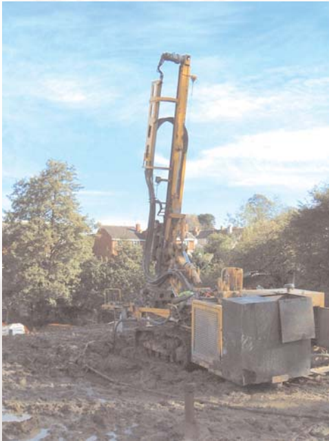
Figure 1 - Drilling the grid
