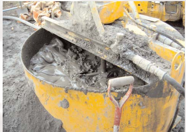
Figure 5 - Feeding the mixer with PFA
