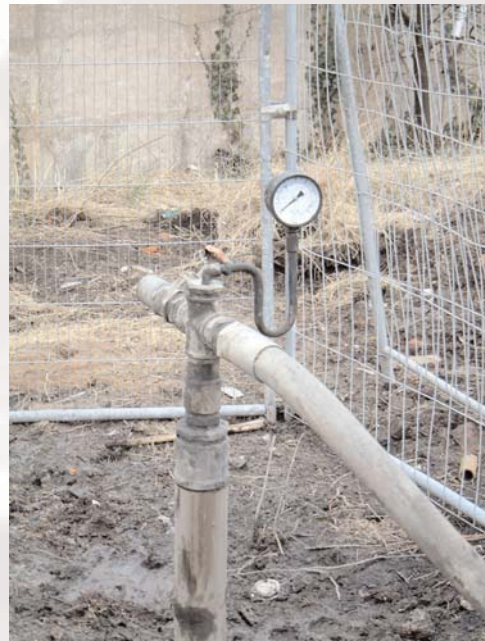
Figure 2 - A grout injection point
