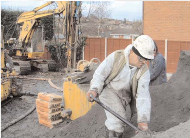
Figure 5 - Feeding the mixer with PFA
